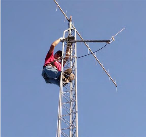
Removing the J-Pole Antenna
