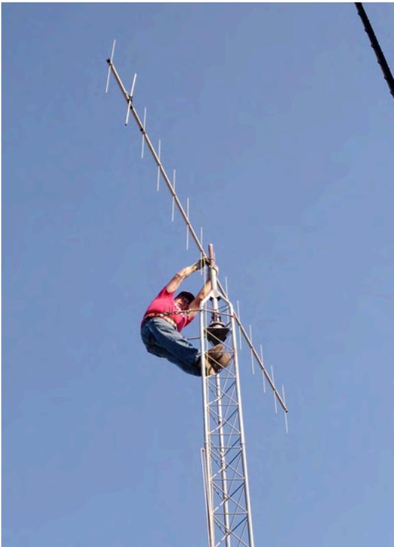
Removing the Beam Antenna
