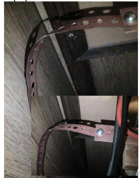
I mounted my Power pole distribution box securely to the bracket and ran short lengths of braid from the
